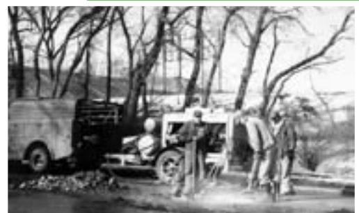
Water Main Repair (ca. 1954)
