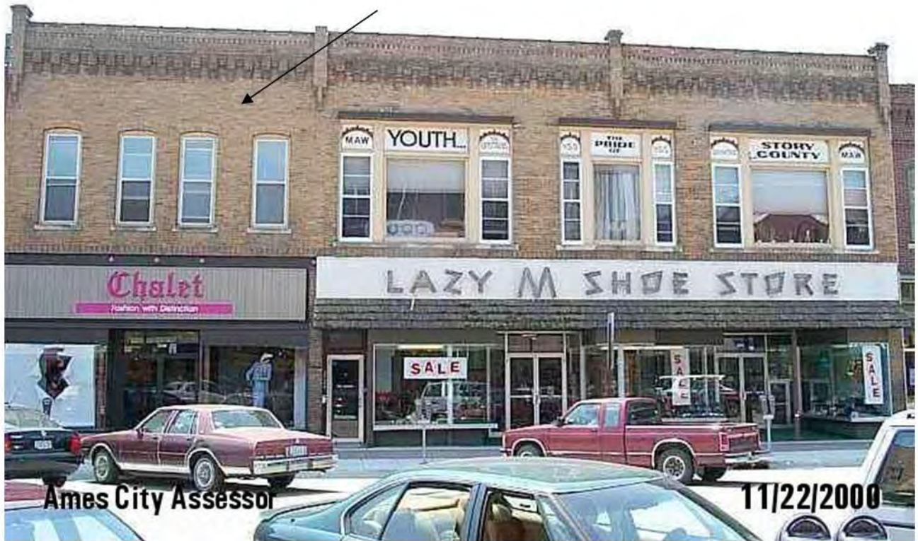
230 Main Street before door and window replacement. Photo taken 11/22/2000.
