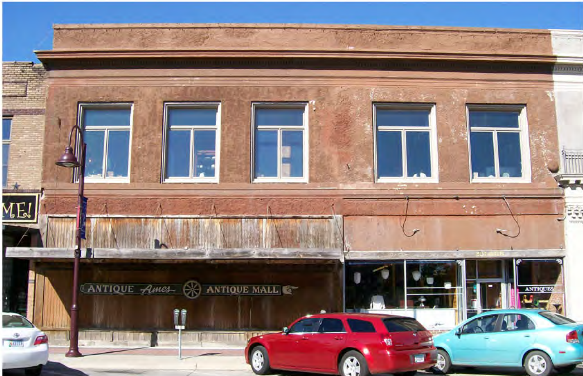
203 Main Street after upper window replacement. Photo taken June 1, 2006.
