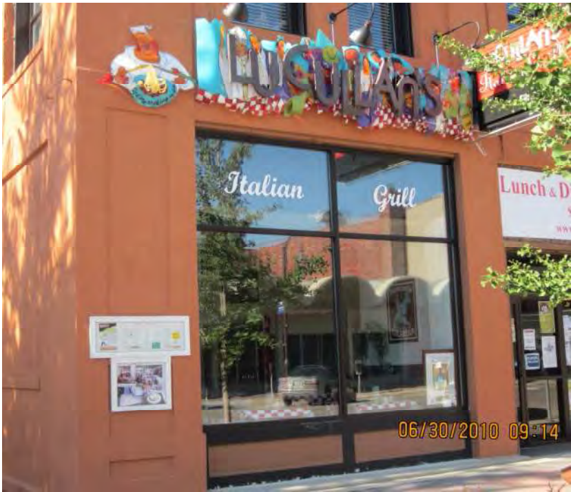
400 Main after replacement of display window, entrance and sign
