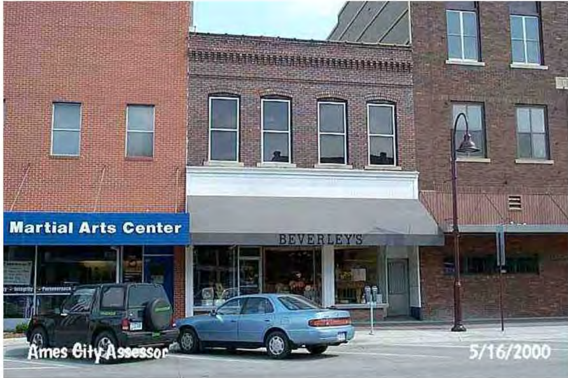
229 Main Street before display window and lighting replacements. Photo taken 5/16/2000.
