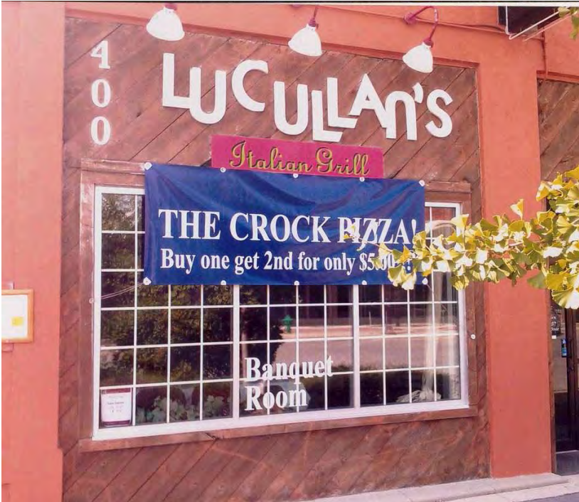
400 Main before façade improvements
