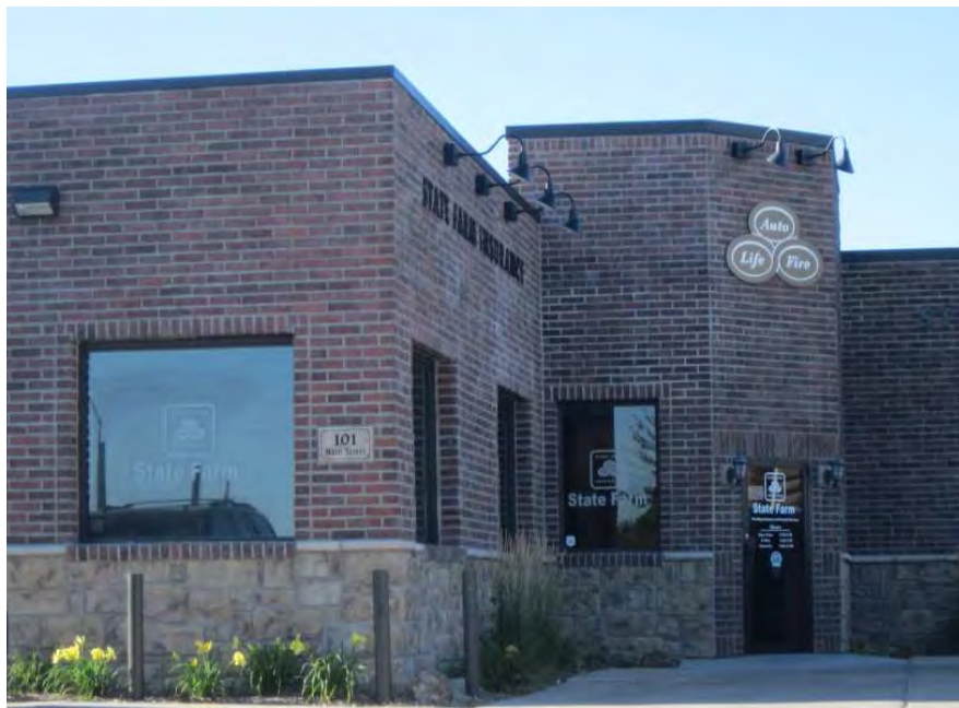
101 Main after parapet reconstruction, masonry veneer, signs, and lighting.
