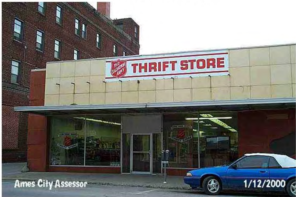
411 Kellogg Avenue before façade and display window replacements. Photo taken 1/12/2000.
