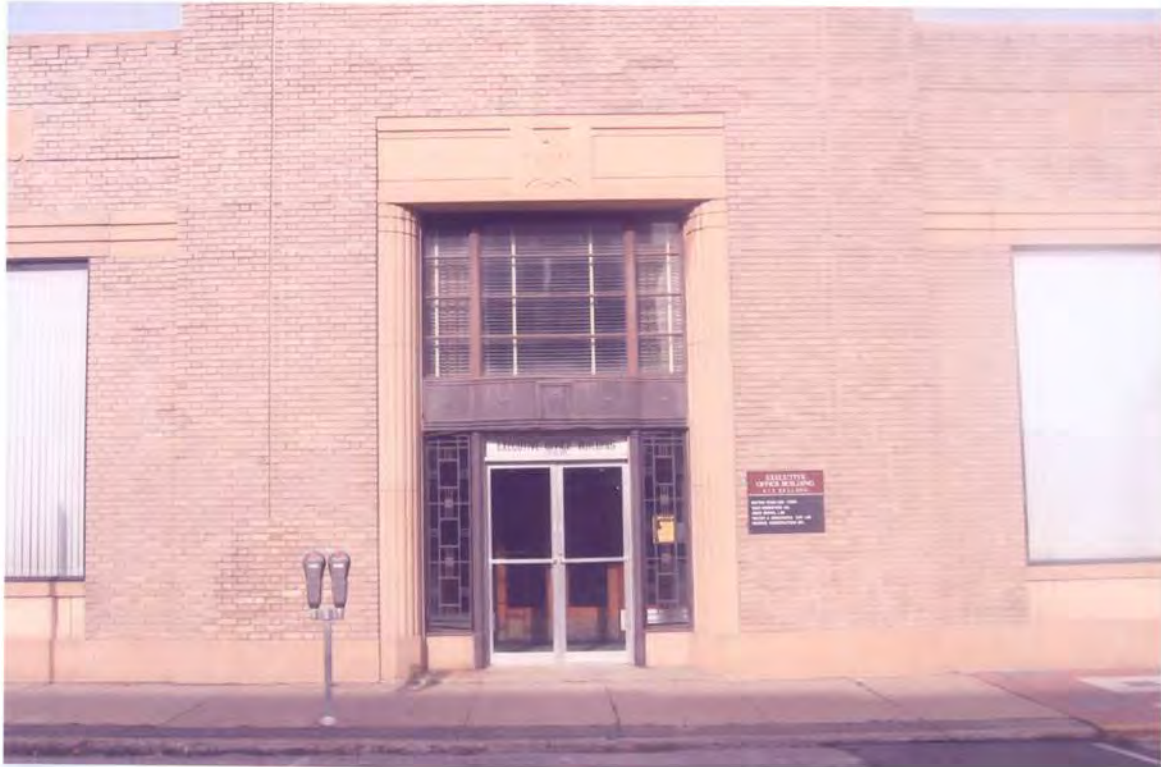
413 Kellogg Avenue main entrance before grant.
