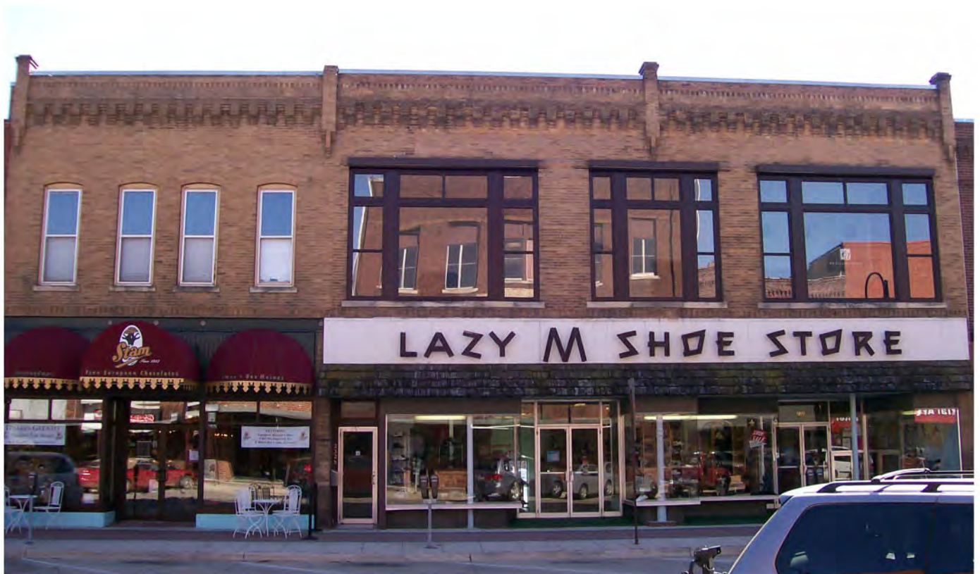
230 Main Street before door and window replacement. Photo taken 6/12/2008.
