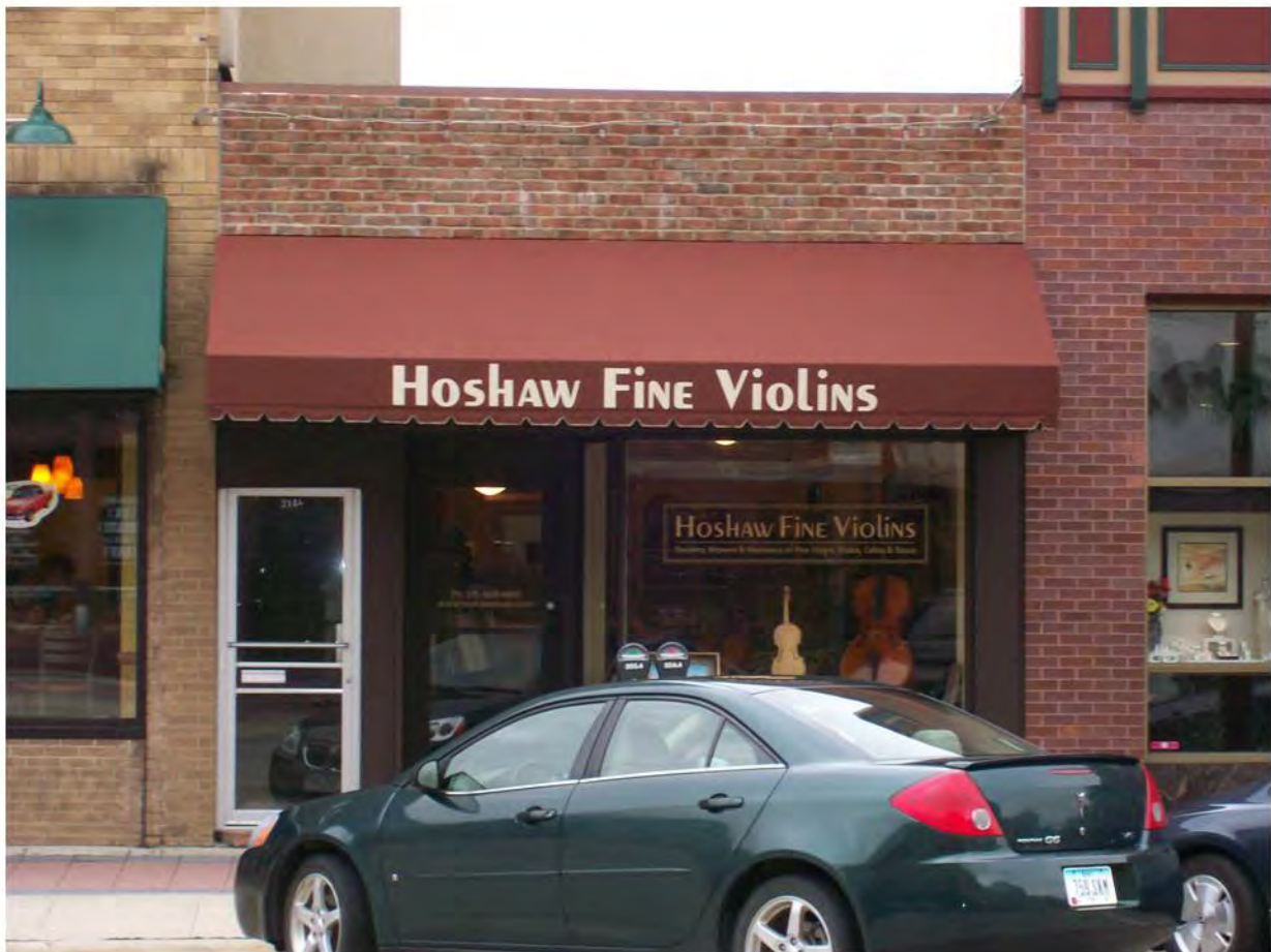
218 Main Street after façade, window, and awning replacement. Photo taken 6/12/2008.
