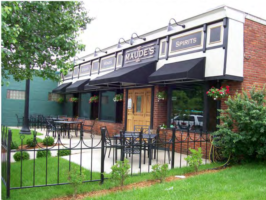
547 Main Street after façade and window replacement. Photo taken 6/12/2008.
