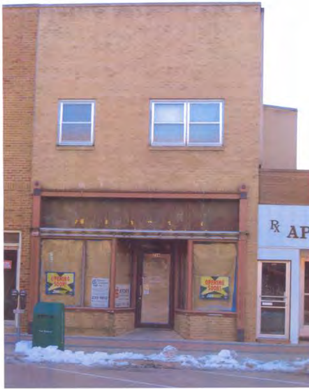
216 Main Street before façade, window, and awning replacement. Photo taken 11/2000.
