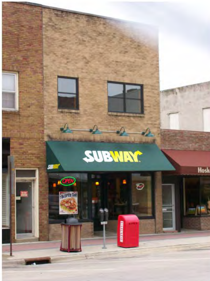
216 Main Street after façade, window, and awning replacement. Photo taken 6/12/2008.
