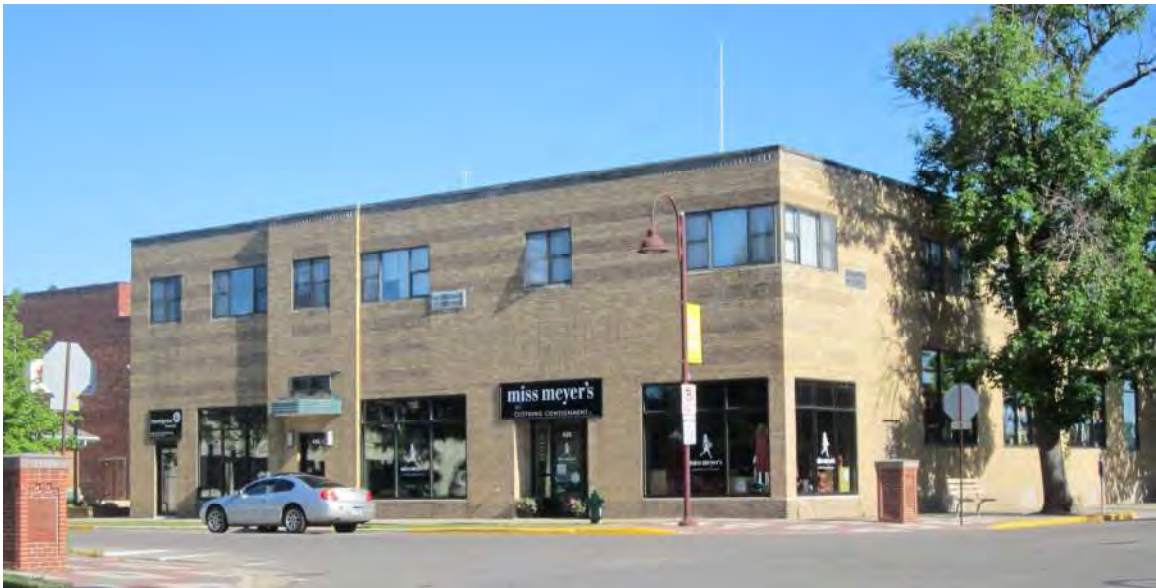
426 Fifth after replacement of windows, and entrances, masonry restoration and signs
