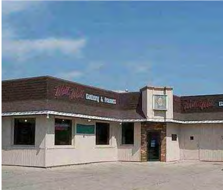
101 Main before renovation
