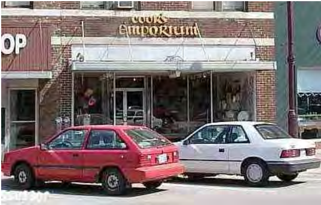
313 Main before façade improvements
