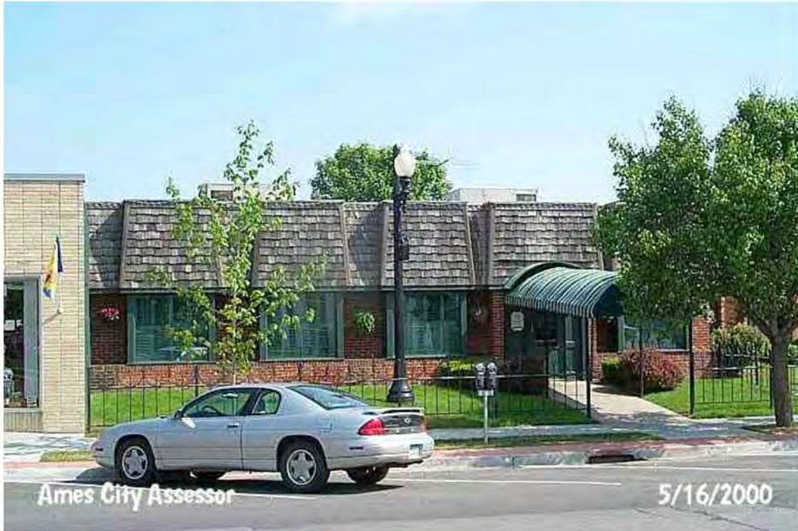
547 Main Street before façade and window replacement. Photo taken 5/16/2000.
