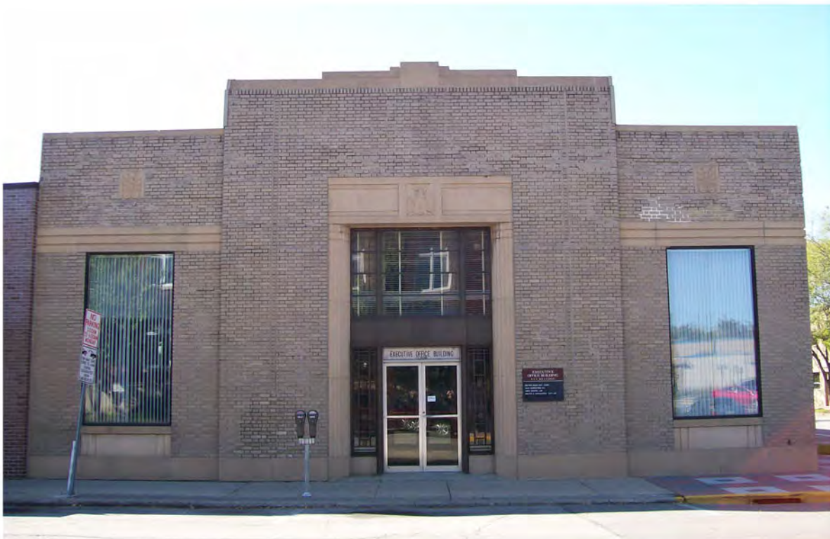
413 Kellogg Avenue after doorway and display window replacement. Photo taken 6/12/2008.
