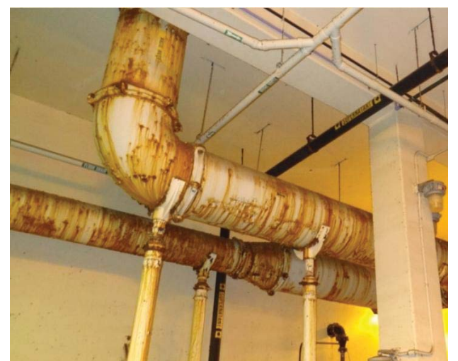
Ames WPCF Condition Assessment
