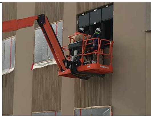
Second floor windows being installed.
