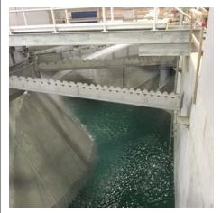
Solids Contact Unit No. 3 being filled on February 24, 2017 to conduct a leak test.
