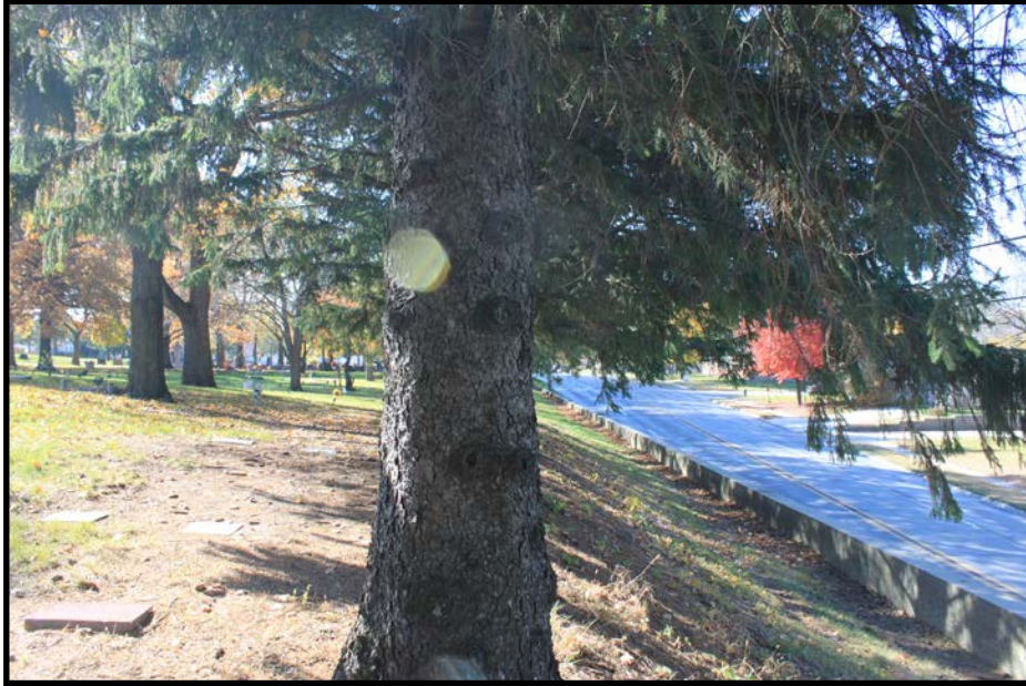
Figure 46. 13th Street wall, view to the west.
