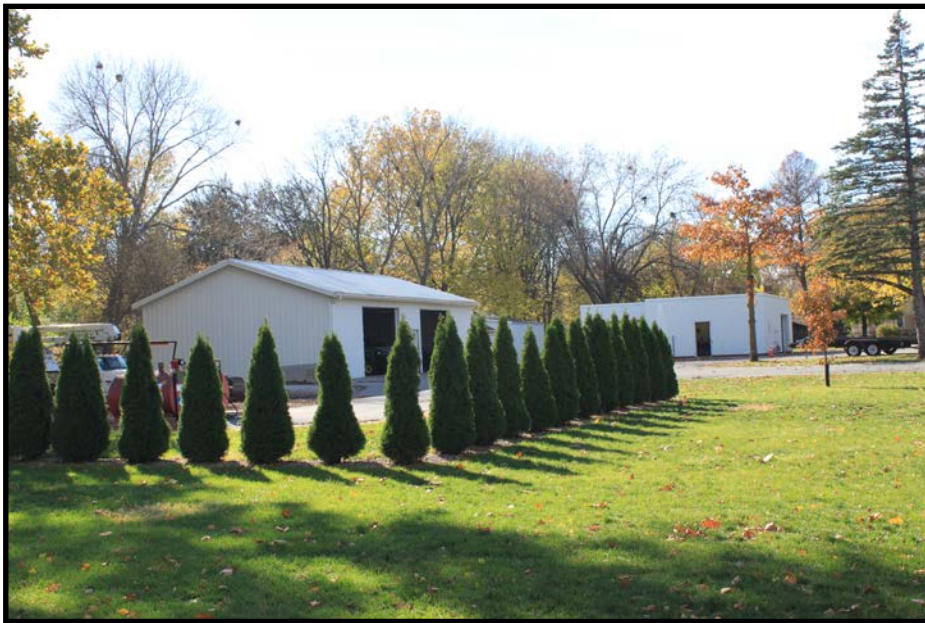
Figure 47. Garages and Break Room, view to the west.
