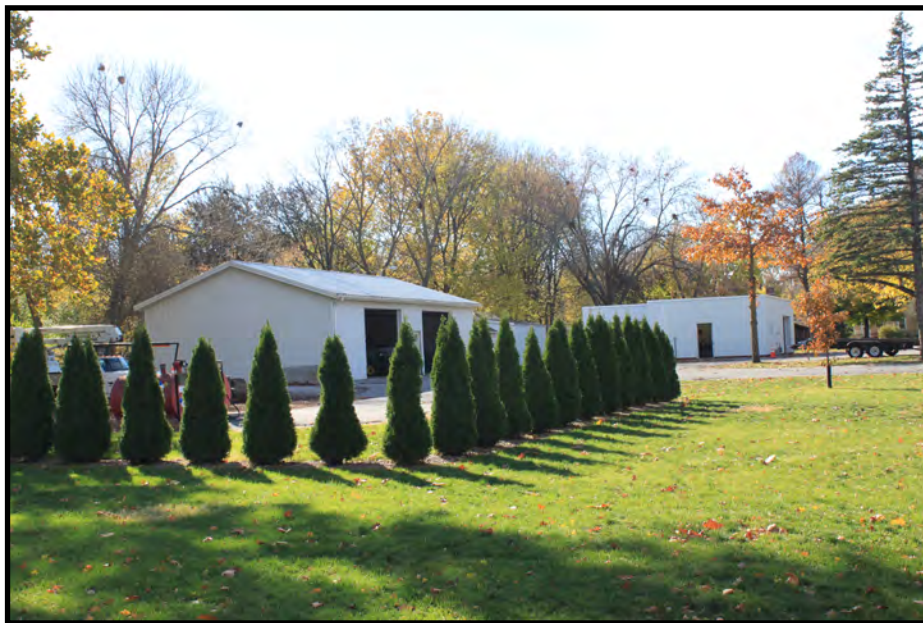
Coverage of Ames Municipal Cemetery, Garages and Break Room, view to the west
