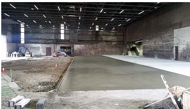
Above are more photos of the replacement work for the tipping floor at Resource Recovery
