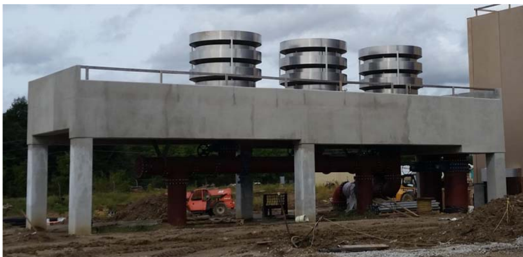
Aerators on September 16, 2016
