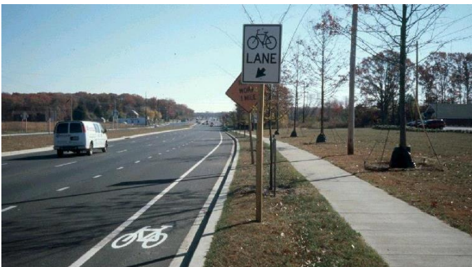
Context is important in Complete Streets design. Although an attempt at improving conditions for walking and biking have been made in example streets on the left (from another city), it is probable the street cannot be considered complete. Traffic volumes and speeds are too high for the unprotected bike lane to serve most people bicycling.
