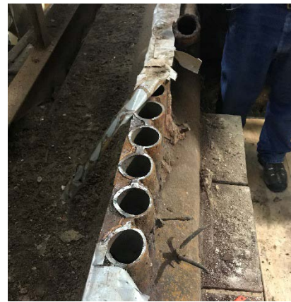
Figure 5 Lower Wall North Side Header
