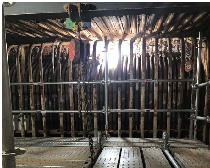
Figure 1 Unit 7 Front Side of Generating Bank tubes
