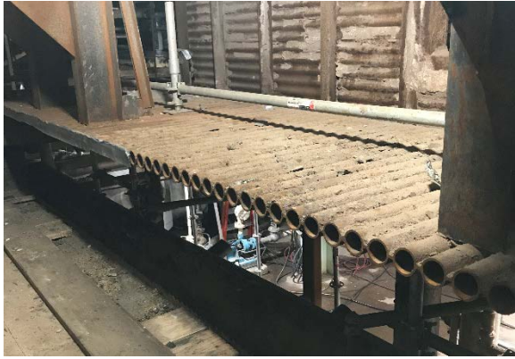
Figure 2 Bottom Tubes on Rear Wall
