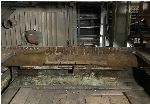
Figure 4 Unit 7 Lower Wall North Side Header
