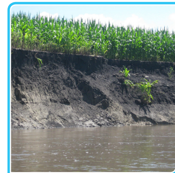
Streambank erosion near farm field. Source: Iowa Learning Farms
