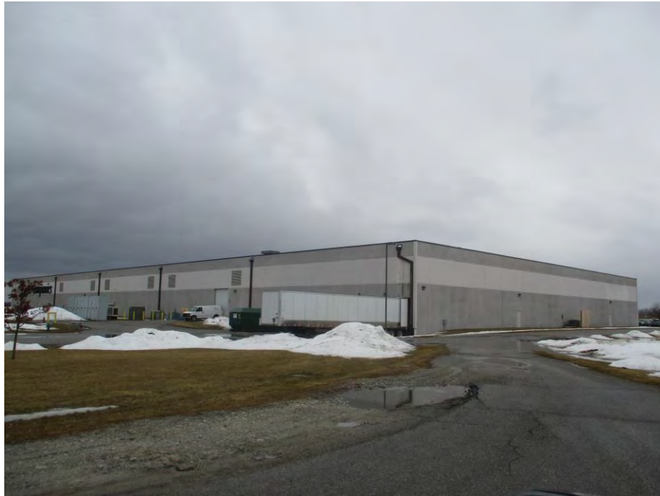
Northwest Building Elevation - Warehouse
