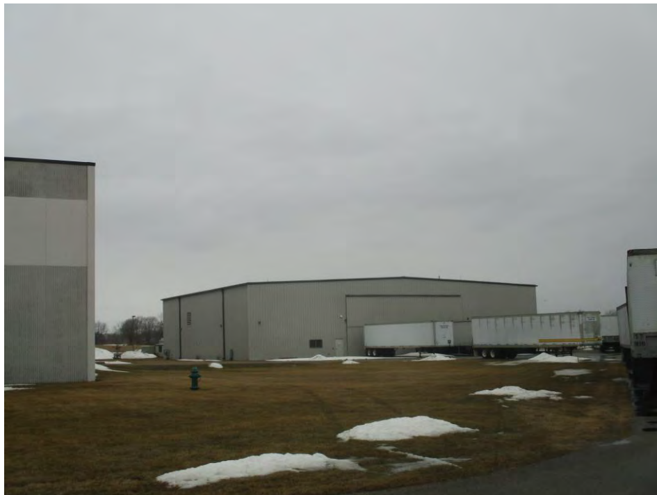
Southeast Building Elevation – Storage Hangar
