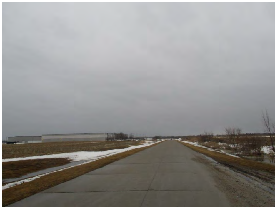
Looking East Along Access Road
