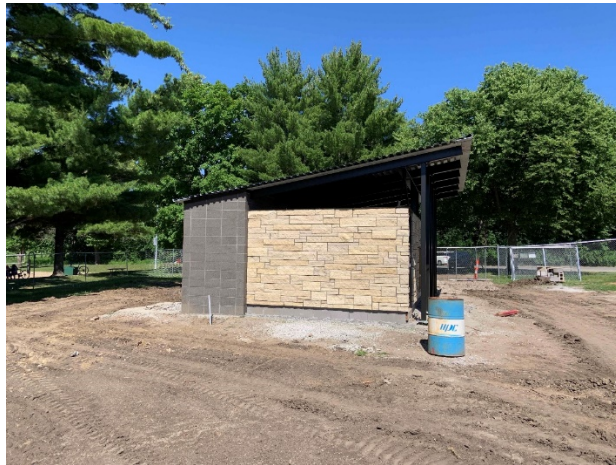
New Inis Grove restroom north of tennis courts
