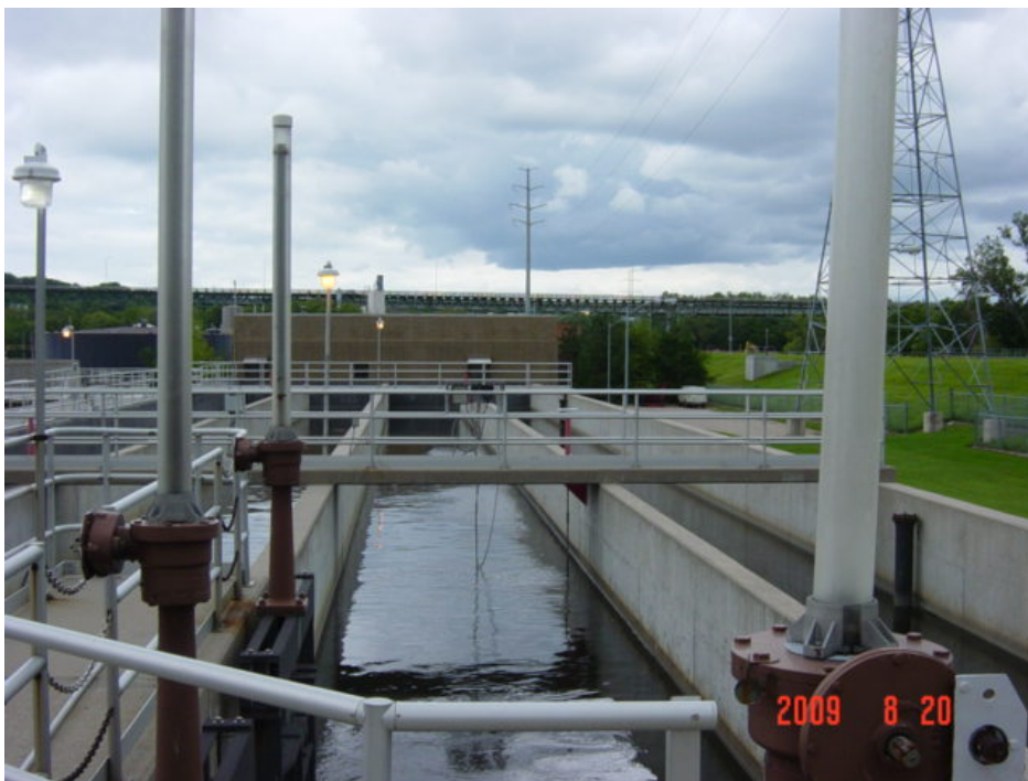
Chlorine Contact Basin – Omaha WWTP
