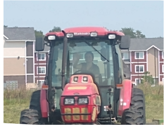
Kayley Barrios Lain spent a recent afternoon on a tractor at the SunSmart Ames site on Airport Road. She focused on knocking down wild vegetation to prepare the property for the solar installation this fall.
