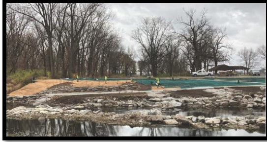
Low Head Dam Nearing Completion
