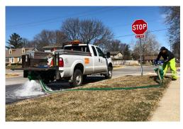
Checks for closed valves and weak flows in the water system
