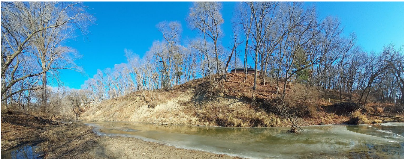
Figure 1: View of the till bluff east bank of loway Creek in Brookside Park from approximately station 11+00 (see Figure 2). Flow is from left to right.
