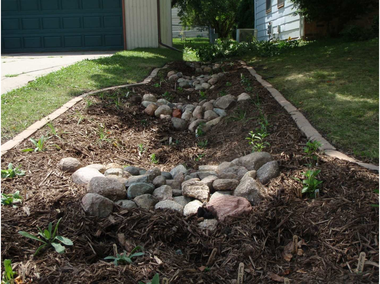
Completed and planted bioretention cell on Emerson Drive.
