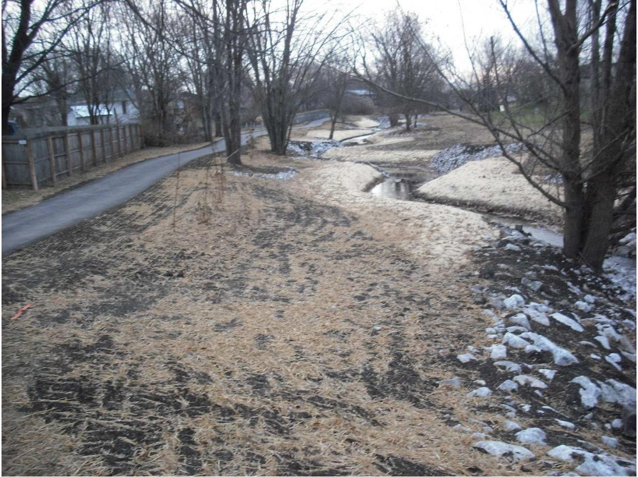
Post-construction view of the restored stream channel shows mature trees salvaged, the two-stage channel and near-stream areas seeded and planted with native vegetation.
