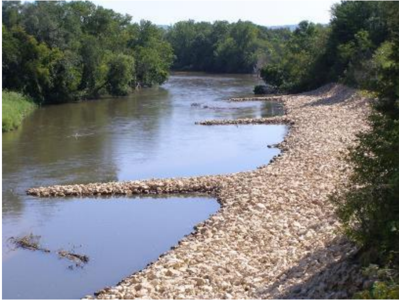
At installation of stream-barbs
