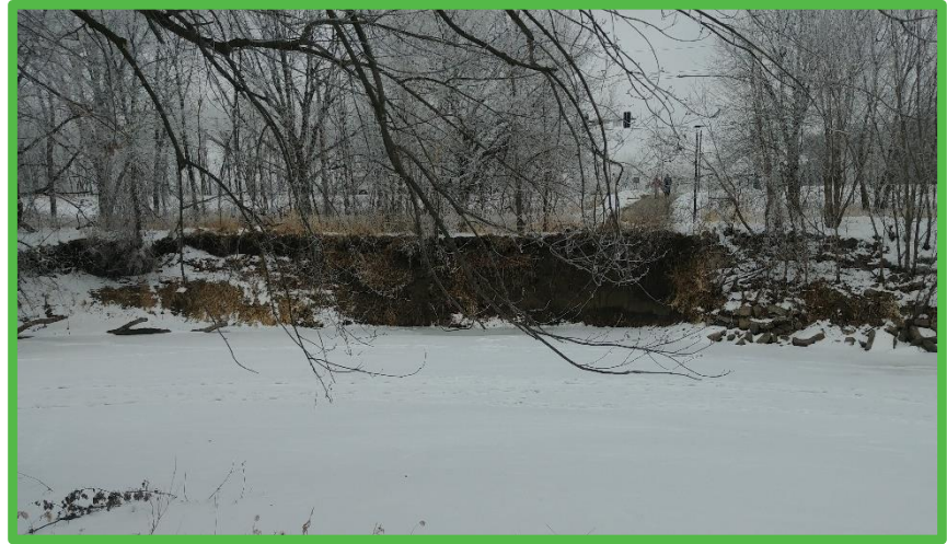
Bank Erosion at Path North of Pedestrian Bridge
