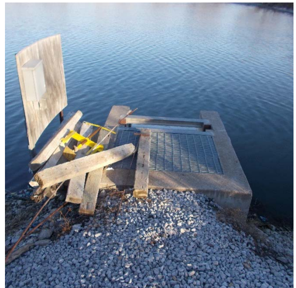
Photo 12: 2020 Ash pond outlet structure
