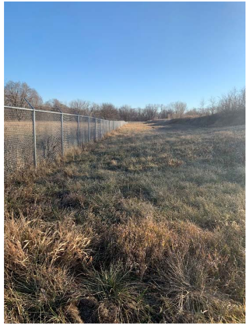
Photo 34: 2020 Chain link fence installed around perimeter of the ash pond property.
