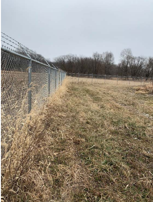
Photo 33: 2019 Chain link fence installed around perimeter of the ash pond property.
