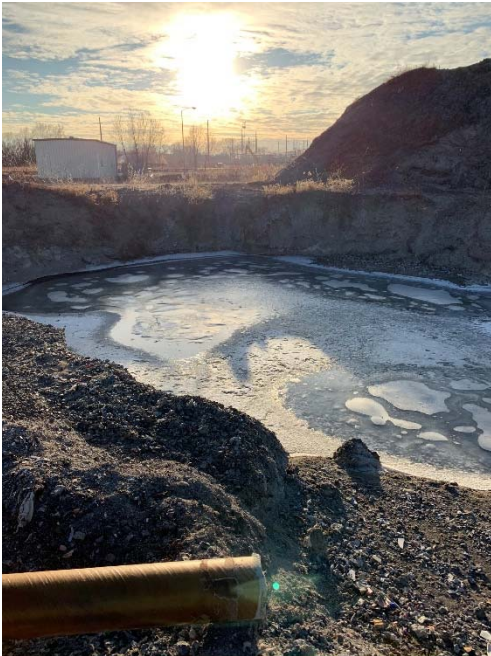
Photo 25: 2019 Ash sluice pipe to West Ash Pond Receiving Ditch
