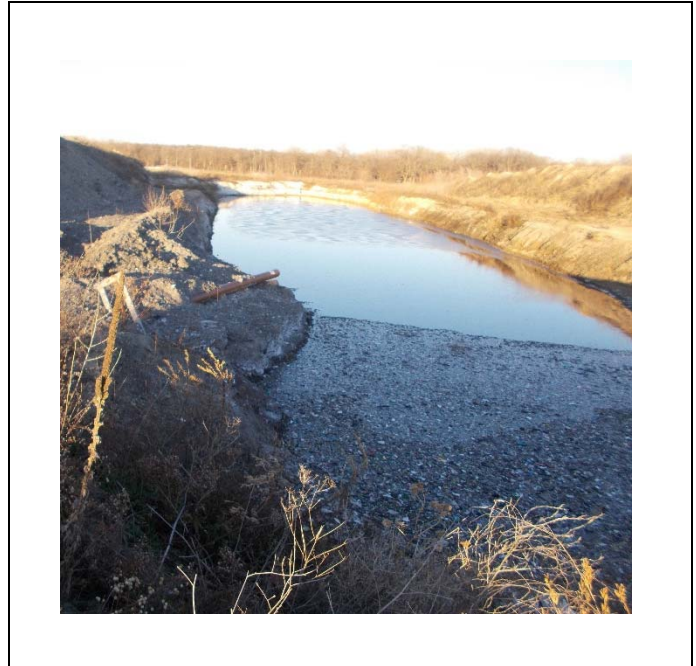
Photo 2: 2020 East Ash sluice pipe to Ash Pond Receiving Ditch
