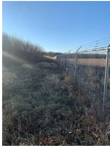
Photo 10: 2020 Outside slope north embankment viewing west.
