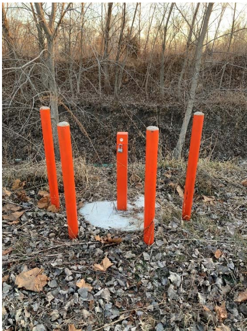
Photo 27: 2019 Typical groundwater monitoring well installed in June 2018.
