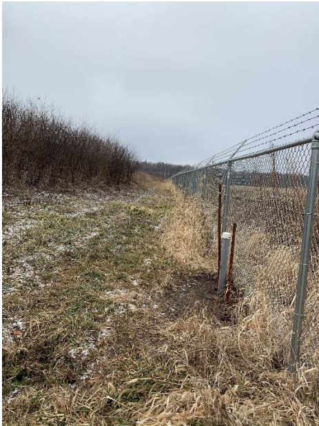
Photo 9: 2019 Outside slope north embankment viewing west.
