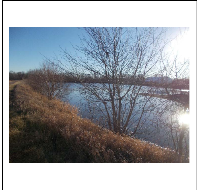
Photo 20: 2020 Example of vegetative growth to be removed on northeast corner of the ash pond.
