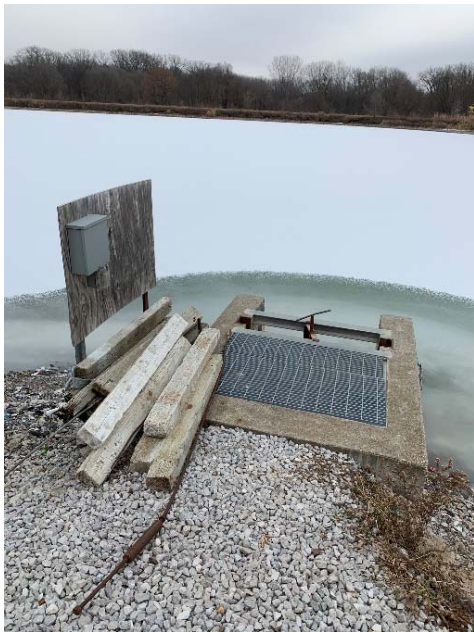
Photo 11: 2019 Ash pond outlet structure
