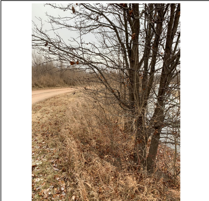
Photo 19: 2019 Example of vegetative growth to be removed on northeast corner of the ash pond.
