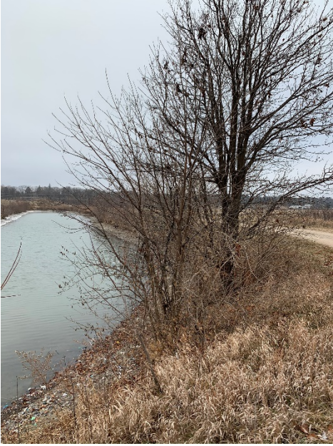
Photo 5: 2019 North dike interior slope view west along ash pond
