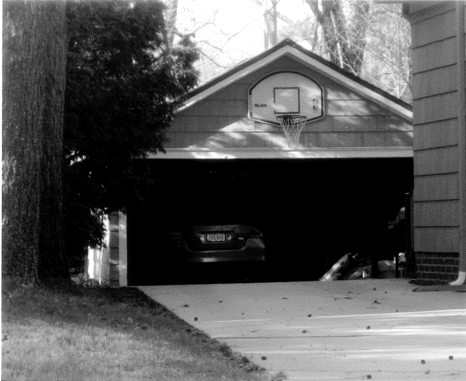
Garage looking north.
