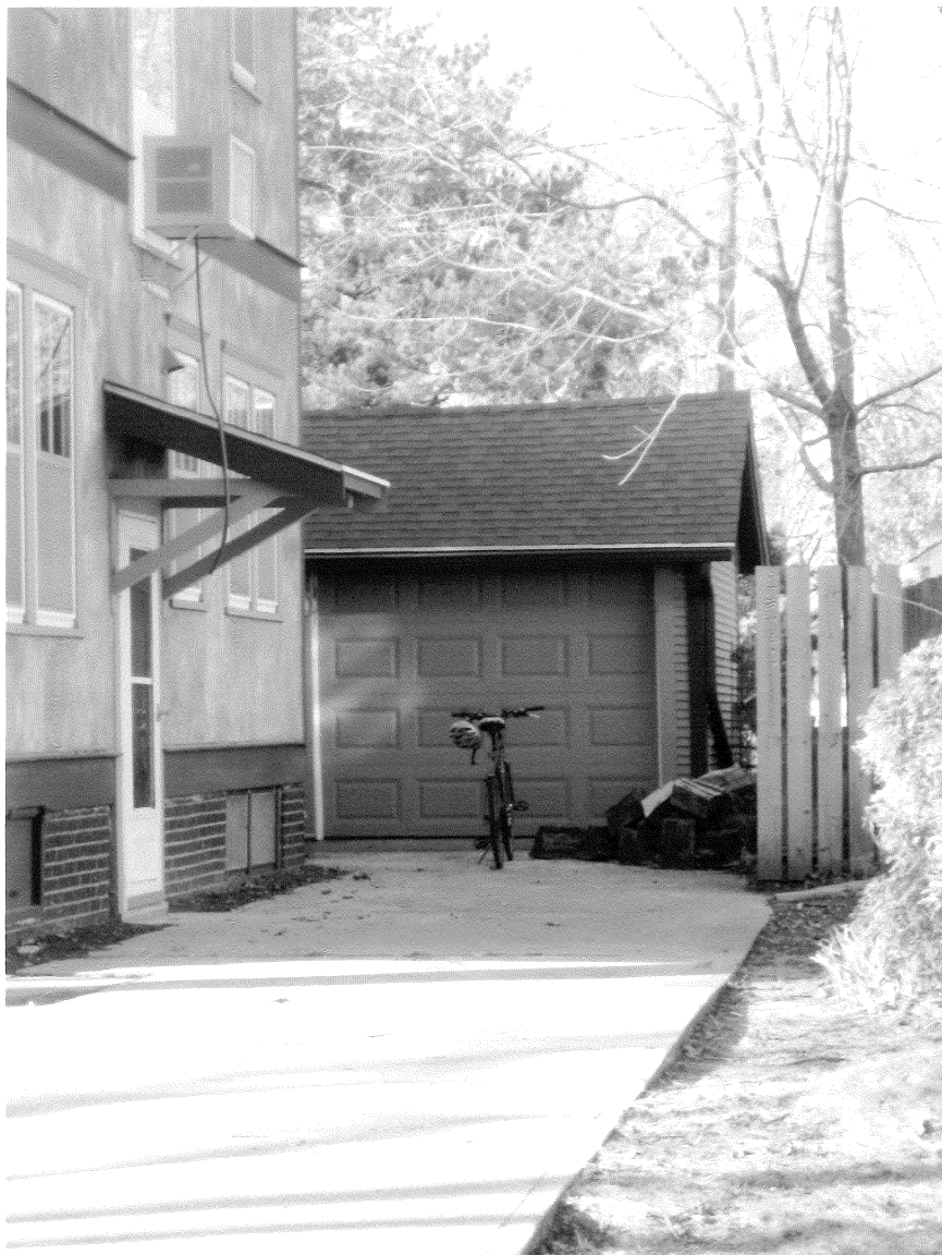
Garage looking north.
