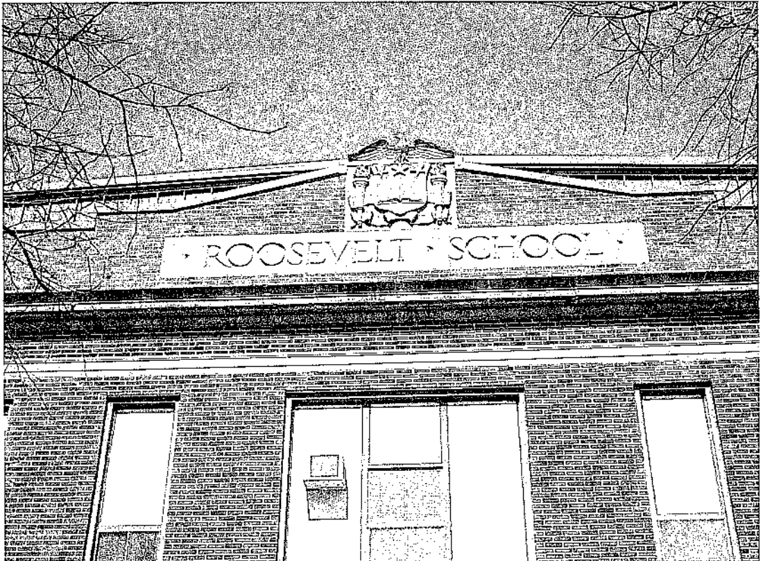
Detail of pediment name plaque and emblem on original Roosevelt School building, View to the North
