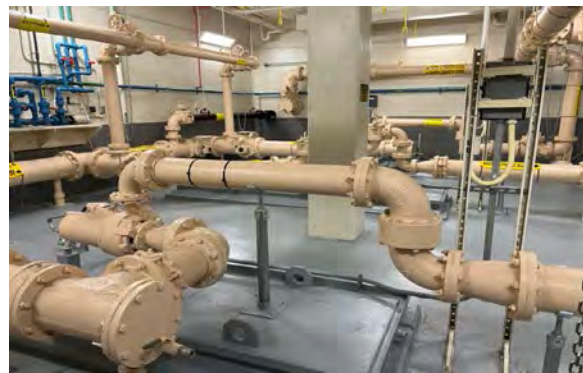
Sludge Pump Building basement after project completion
