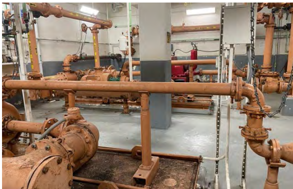
Sludge Pump Building basement prior to the project
