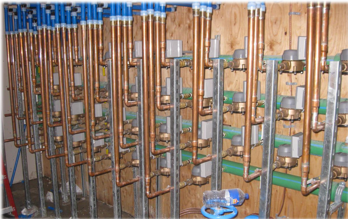
Example of a meter manifold that is typical of a large apartment building.
