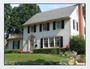
Built in the mid-1920's, this is an excellent example of the Colonial Revival style. Although aluminum siding has been added, there is no apparent loss of ornamentation. Details common to this style are a ridgeboard parallel to the street with side *gables*, end-wall chimney, *pedimented* frontispiece at the entry with wide trim boards on each side. There is an *oriel window* at the east on the first story. Windows have 6/6 glazing. The one story addition to the west was built in the 1970's.
