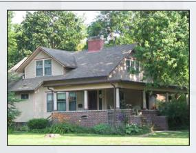
Craftsman influence is seen in this *gabled*-ell cottage evidenced by the wide overhanging eaves, ribbon window, and deep porch. The brick porch has Tuscan columns and a flat roof with closed *sof-fit*. The front stairs have brick bulkheads with concrete caps. A low-pitched *gabled* roof with a *gabled* side *dormer* define the roof area.
