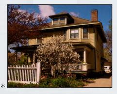
This is a virtually intact example of the American Four Square style. Also called a hipped cottage, it has hipped main roof, hipped *dormers* and also a *hipped roof* on the porch all with flared eaves. The porch has classic columns and a square-spindled railing.
