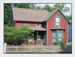
Constructed around 1890, this *gabled*-ell cottage shows us that rich architectural detailing is not only for large elaborate houses. The prominent first story bay window features a paneled bulkhead surmounted with a *cornice* and paired brackets. The windows feature 2/2 glazing. An unusual round window is seen on the front *facade* at the second story. Shaped *lintels* are found over the window openings.
