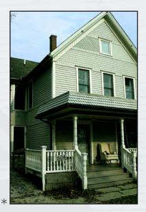
This gabled-ell cottage has many Queen Anne details. Take a look at both the south and west facades. Surface textures include patterned shingles in the gable, narrow diagonal vertical and wood horizontal siding. The fullwidth front porch has been constructed using a historic photo as a guide.
