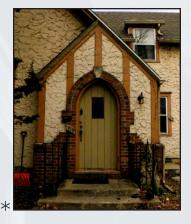
The only Tudor style structure in the district, this style is characterized by a steeply-pitched front *gable* with intersecting side *gable*; half-timbering in the front *gable* and on the entry porch; pointed arched front entryway; 8/1 *glazing pattern* on the windows and roughtextured stucco cladding. The front entry way and door are surrounded by brick with a cast concrete key stone and brick bulkheads.
