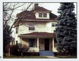
Imagine putting your house together like a jigsaw puzzle! That is exactly how this house was built. This American Four Square is a documented Montgomery Ward Catalog house. Specific styles and details were chosen according to taste and cost and a house was ordered. The pieces came cut, carefully labeled and numbered for the homeowner (or a contractor) to put together.
