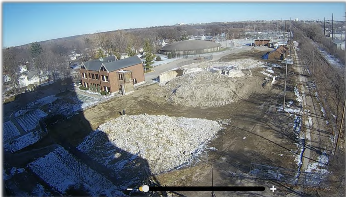
Demolition of the old Water Plant, as seen from the Power Plant
