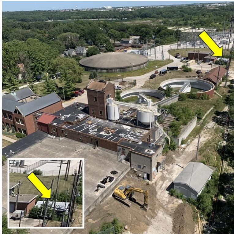
*Photo (8-26-2022) of the old Water Treatment Plant at the start of demolition. The storage building with the unknown remnants of a pump station below is marked with an arrow.*
