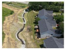
methods for stream restoration with a main feature being the relocation of 200 feet of the stream to the north away from the homes. The channel was raised, the stream banks were flattened, and rock step pools were installed to allow for the channel to be flattened, reducing erosivity of the waterway. Native vegetation was then planted along the stream banks.
